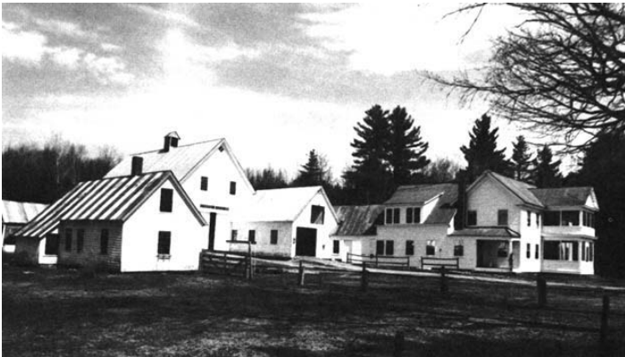
Figure 40 A connected farm complex in Fryeburg, Maine.
