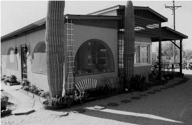
Figure 77 Double-shed additions to trailer outside Phoenix, Arizona.
