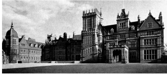
Figure 25 Robert Kerr, Bear Wood, near Wokingham, Berk- shire (1865–74), exterior.
