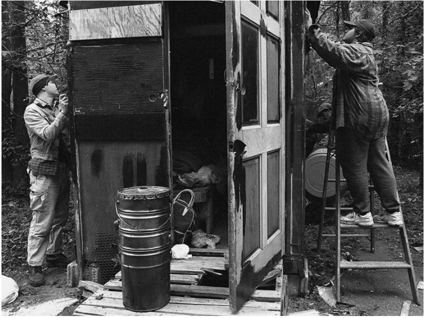
Figure 83 Construction of Mad Houser hut, Atlanta, Georgia, c. 2002.
