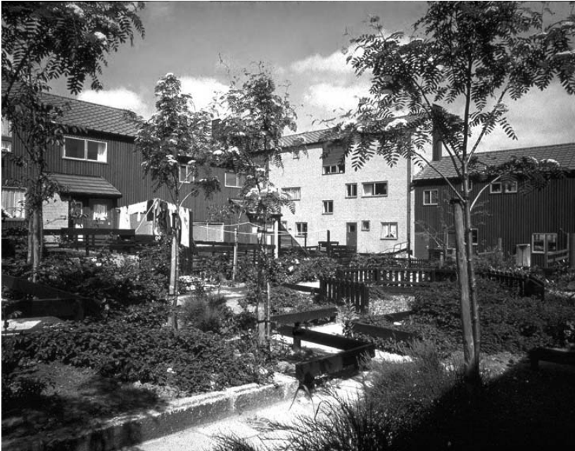
Figure 61 Byker Wall development, Janet Square, 1971–2.
