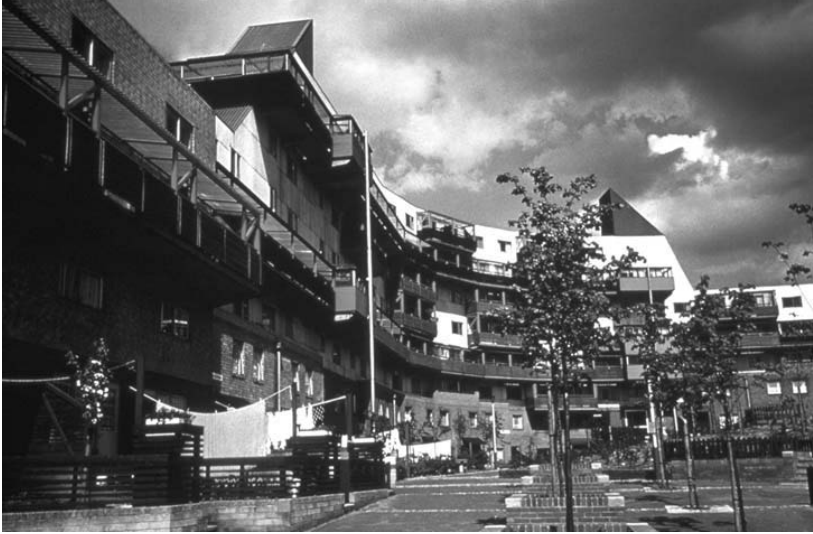
Figure 60 Ralph Erskine, Byker Wall development, Newcastle-upon-Tyne, 1969–81, view of inner face of wall.
