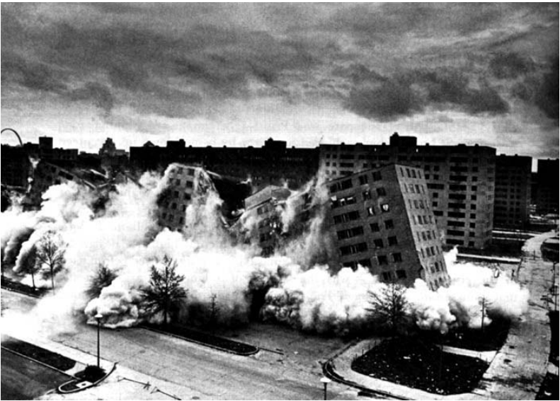
Figure 69 Pruitt-Igoe housing being demolished in 1972
